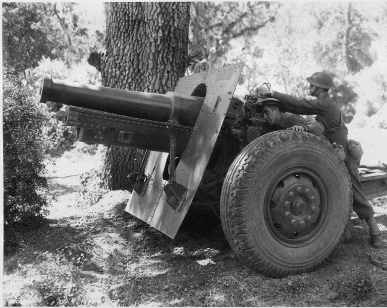
Sgt. James B. Aets uses a quadrant to determine the elevation of the 155mm M1918A3 Schneider, while Cpl. Charles J. Hines sights on the aiming stake, while training stateside in 1942 (US Army Signal Corps Photo).
