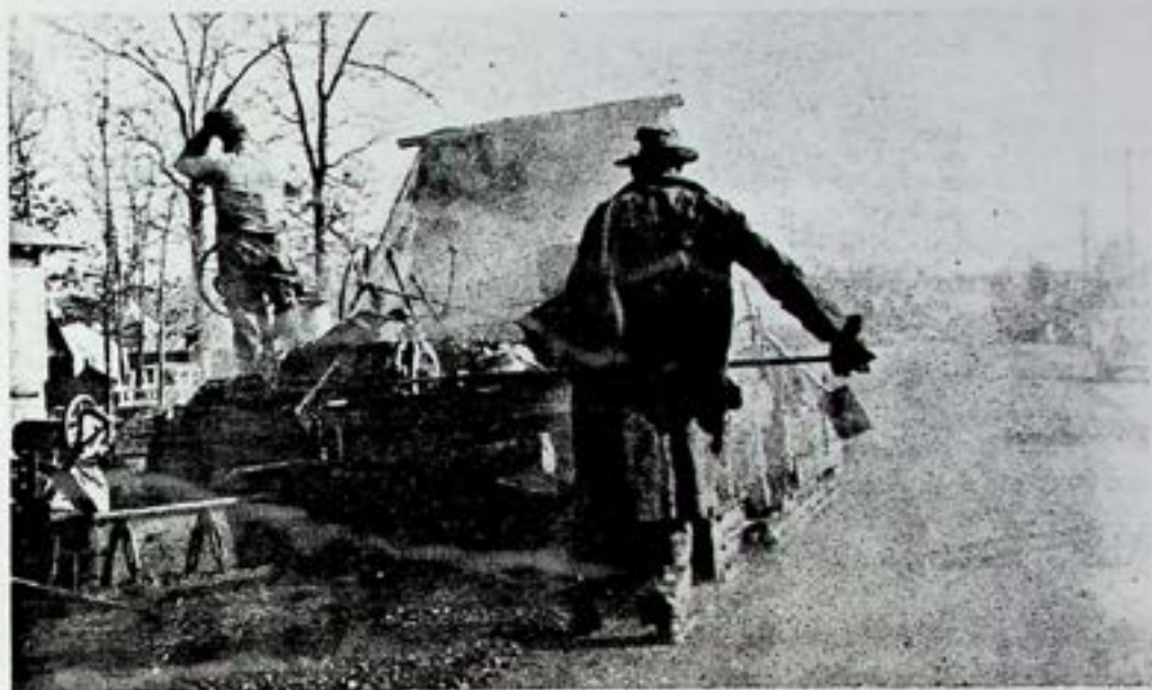
PLACING HOT ASPHALTIC CONCRETE
