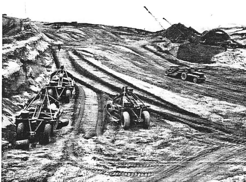
American troops landed on Amchitka in January 1943. A month later, fighters were operating from the new airstrip, and by March medium and heavy bombers were striking Kiska. Here trucks haul sand for runway foundations. The Japanese never were able to complete runways at Kiska and Attu.
